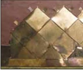
**Chatel Real Estate**—2113 N St., NW, Washington, DC. Replaced the built-in gutters, restored the structural cornice and replaced the copper shingles on the mansard roof. Insert shows new copper shingles that will be installed.
