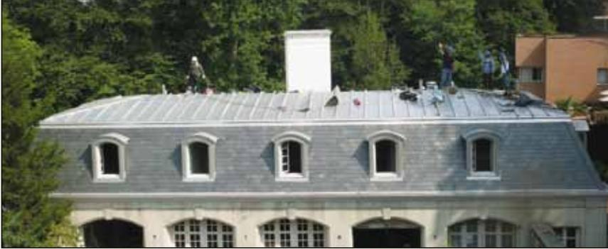
**Belgian Ambassador's Residence:** 2300 Foxhall Rd., NW—Installing new Buckingham slate, built-in copper gutters and batten seam copper roof as seen in photo to the right. Replicated and installed 15 copper dormers and window trim for Whiting Turner Construction Company.
