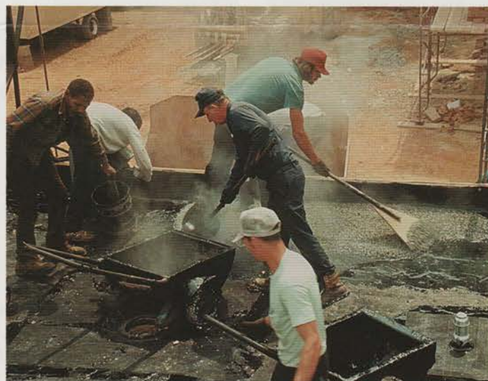
Early Jones (center) leading his built-up-roof crew.
