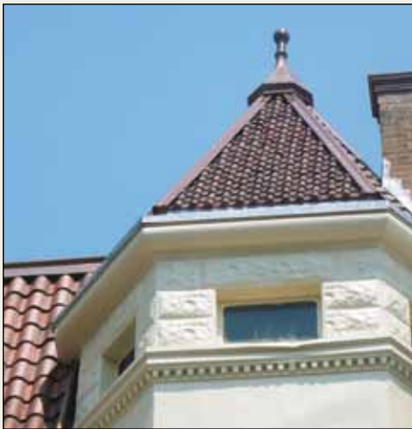
1517 U Street, NW , Washington, DC. Repoint brick joints and limestone, repaint all wood and cornice. Relay tile, new lead-coated copper.
