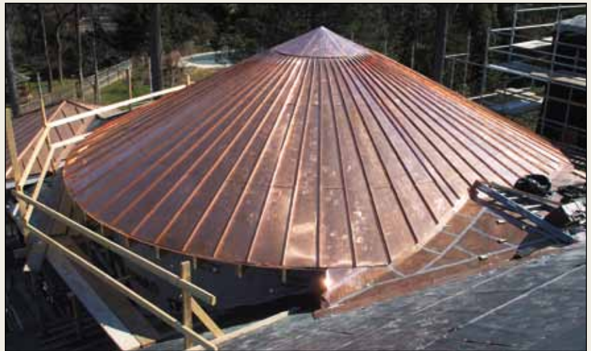
7209 Arrowood Road , Bethesda, MD. General Contractor: Carl Petty & Associates. New slate and standing seam copper roof on dome.
