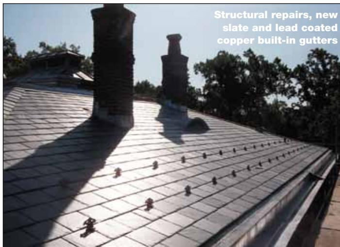
Structural repairs, new slate and lead coated copper built-in gutters
