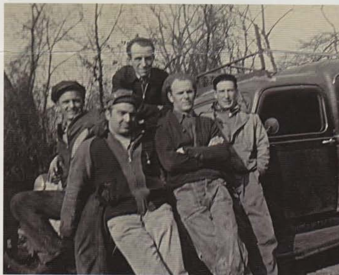
Jack Wagner, Sr. (right) with roofing crew in front of the “Flying Enterprise” ’47 Dodge. The photo probably was taken around 1948.
